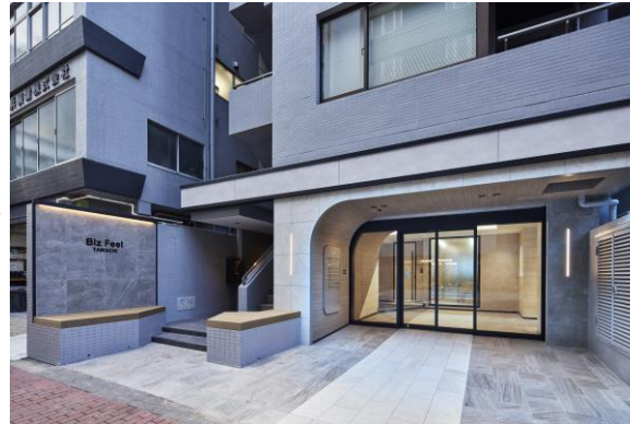
Parking area was converted into an office space.
