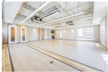
The top floor and a part of the first floor parking lot converted into an office
